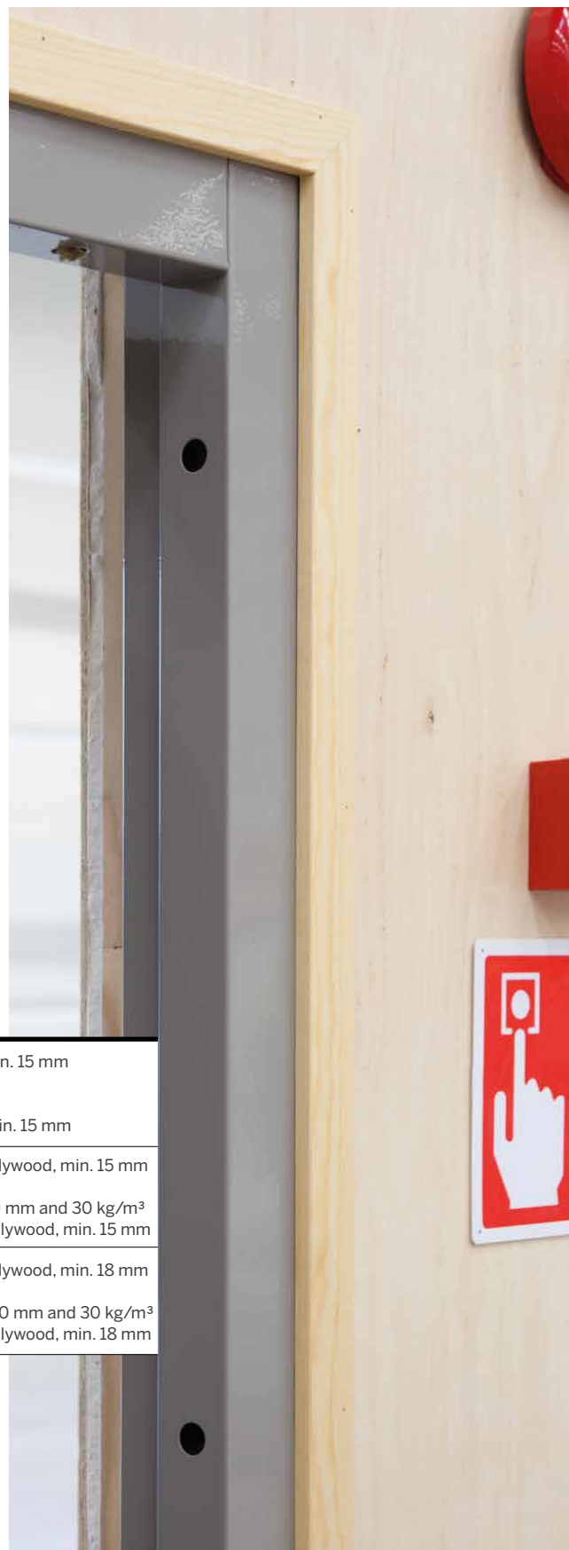
Door opening in a compartment wall
