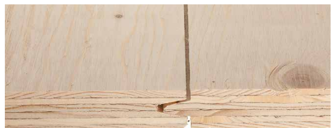
Figure 16. Tongue and groove (TG) joint
