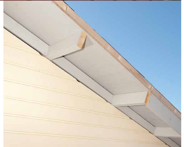
Figure 24. Cantilevers supporting eaves overhang
